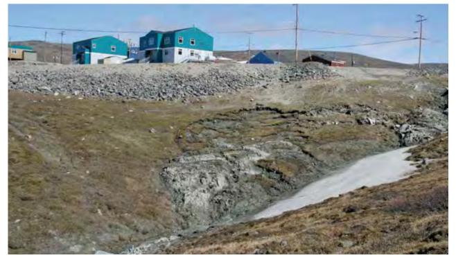
Figure 3. This active layer detachment failure in the village of Salluit occurred in 2005.
