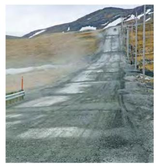
**Figure 6.** Access road to Salluit airport showing important deformations with a succession of thaw settlements.
