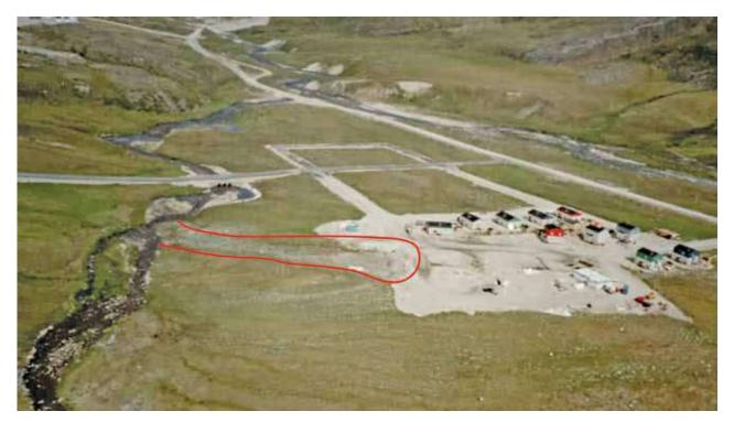
**Figure 7.** This active layer detachment failure in Salluit occured in 1998 and prompted the abandonment of the development project in this sector as well as the removal of 20 houses already built.
